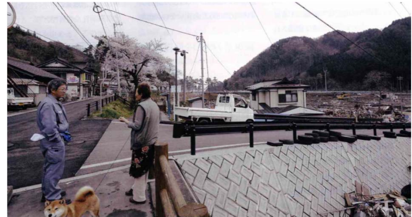
Hongo area of Kamaishi, relocated after 1933 tsunami, damaged again in 2011
