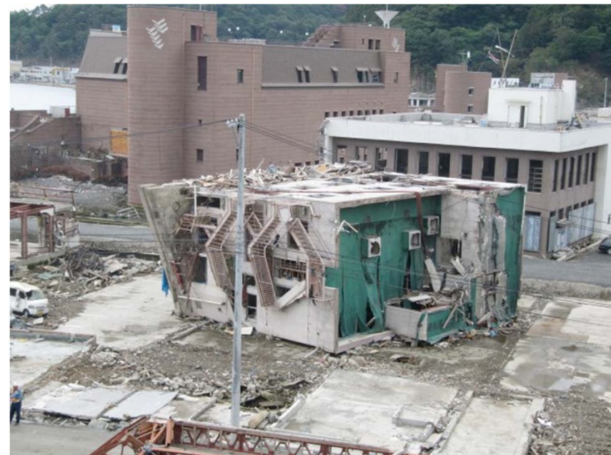
Reinforced concrete building Onagawa town
