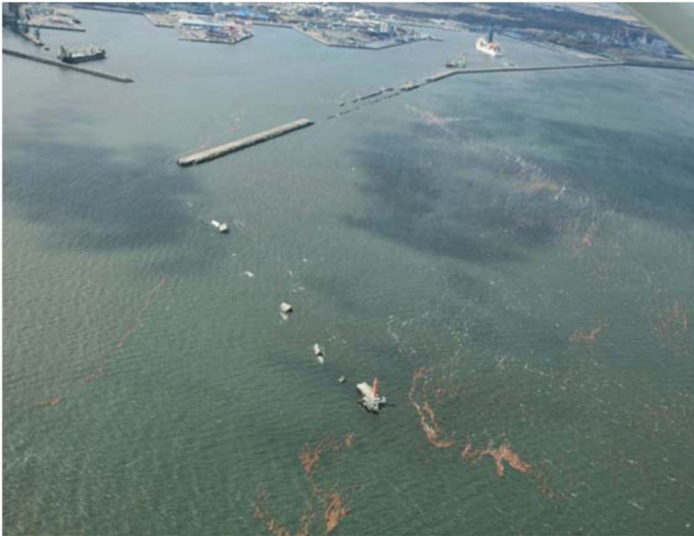
Hachinohe Port Breakwater
