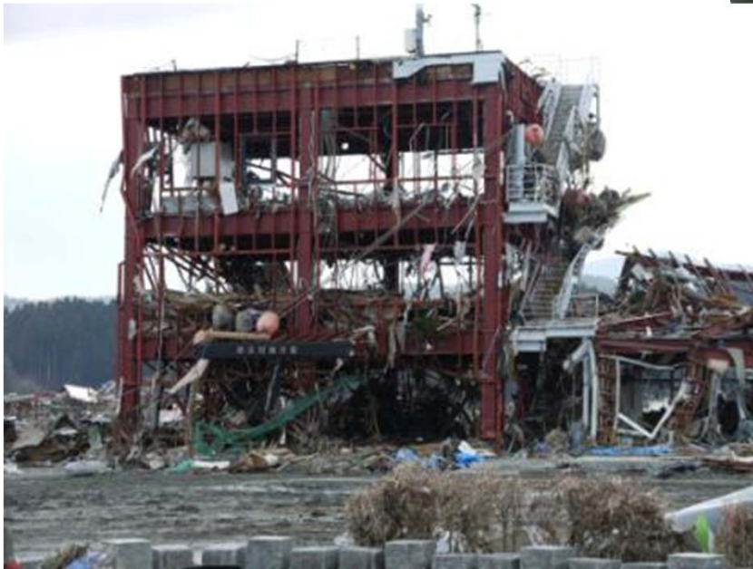
The disaster management center of Minami-sanriku town
