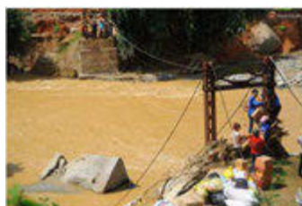
A bridge at Sung Hoang village
