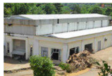
Ngoi San hydro-power after Flash flood
