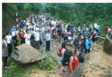
Broken 4D main road.
