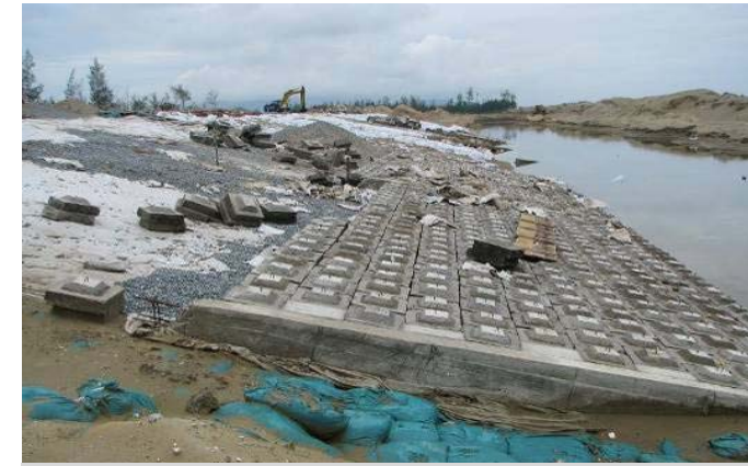
construction of revetment on unstable ground
