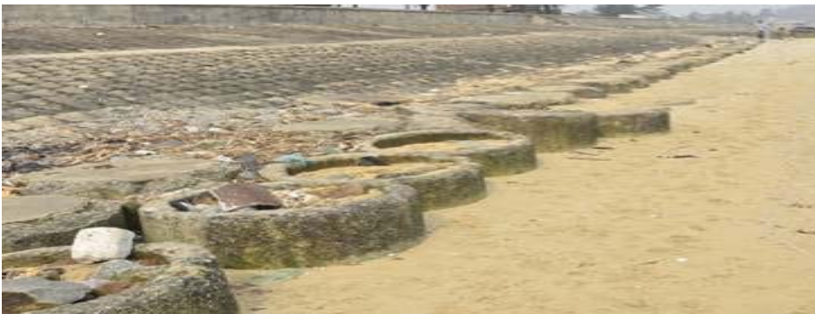
Protect revetment's toe by Cement-pipe
