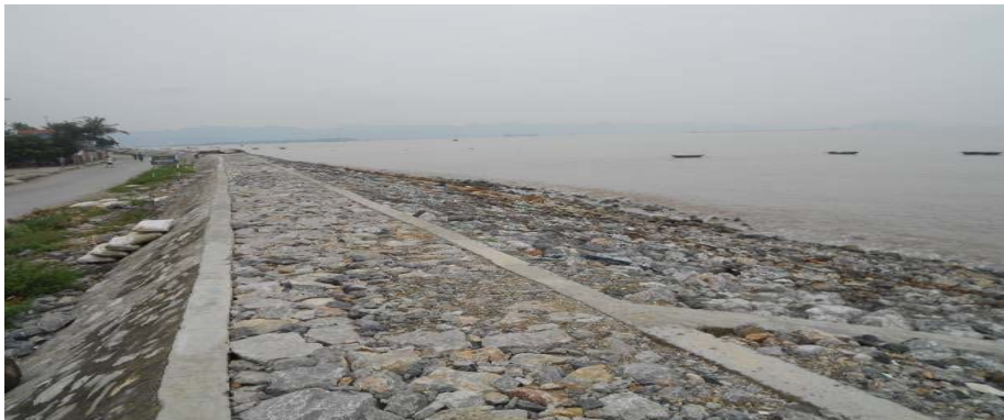
rip-rap revetment with frame
