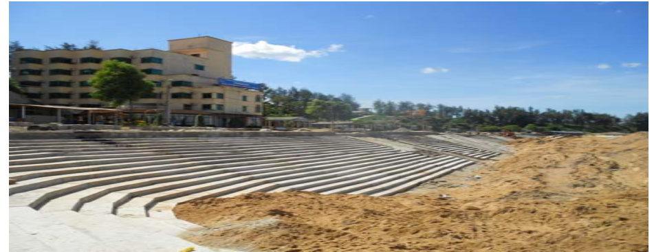
Stepped concrete block revetment
