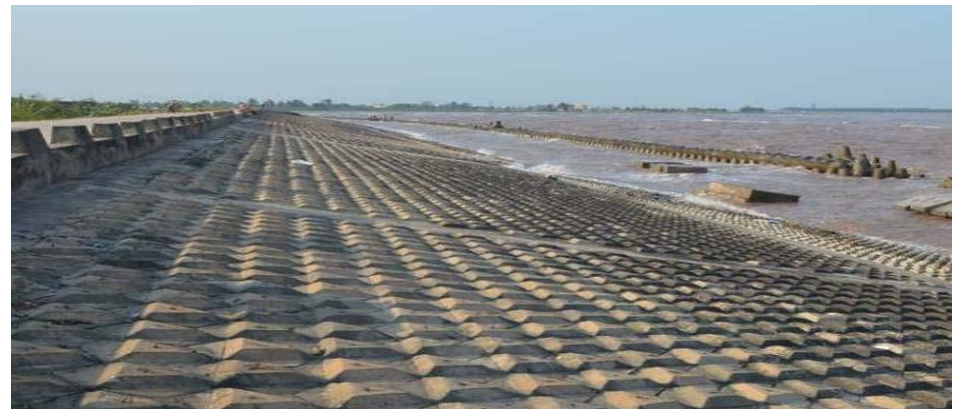
Articulating Concrete Block System
