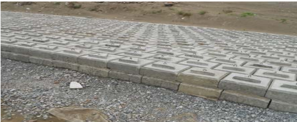
Articulating Concrete Block System
