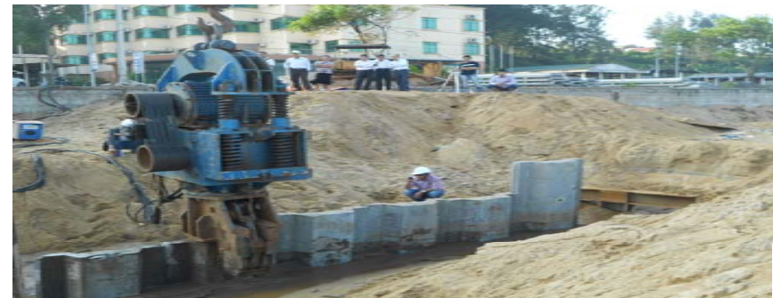
Prestressed concrete piles
