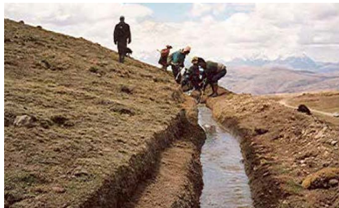
Catcca, Quispicanchi, Cuzco - Infiltration trenches
