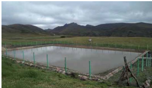
Condebamba, Cajabamba, Cajamarca- Microreservorios
